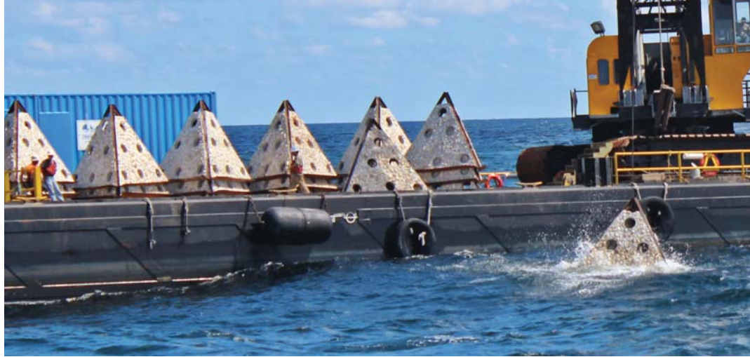
Corpus Christi Nearshore Reef work underway. Being deployed are the new specially-designed pyramid reef elements. Photo, Lisa Laskowski
