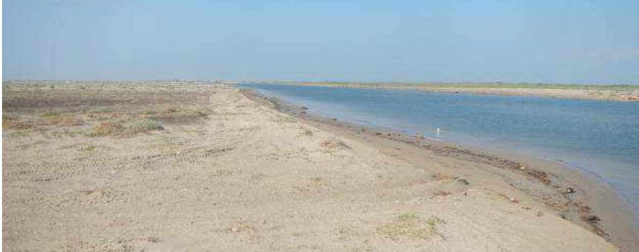
Figure 2. Completed Excavation of Vinson Slough
