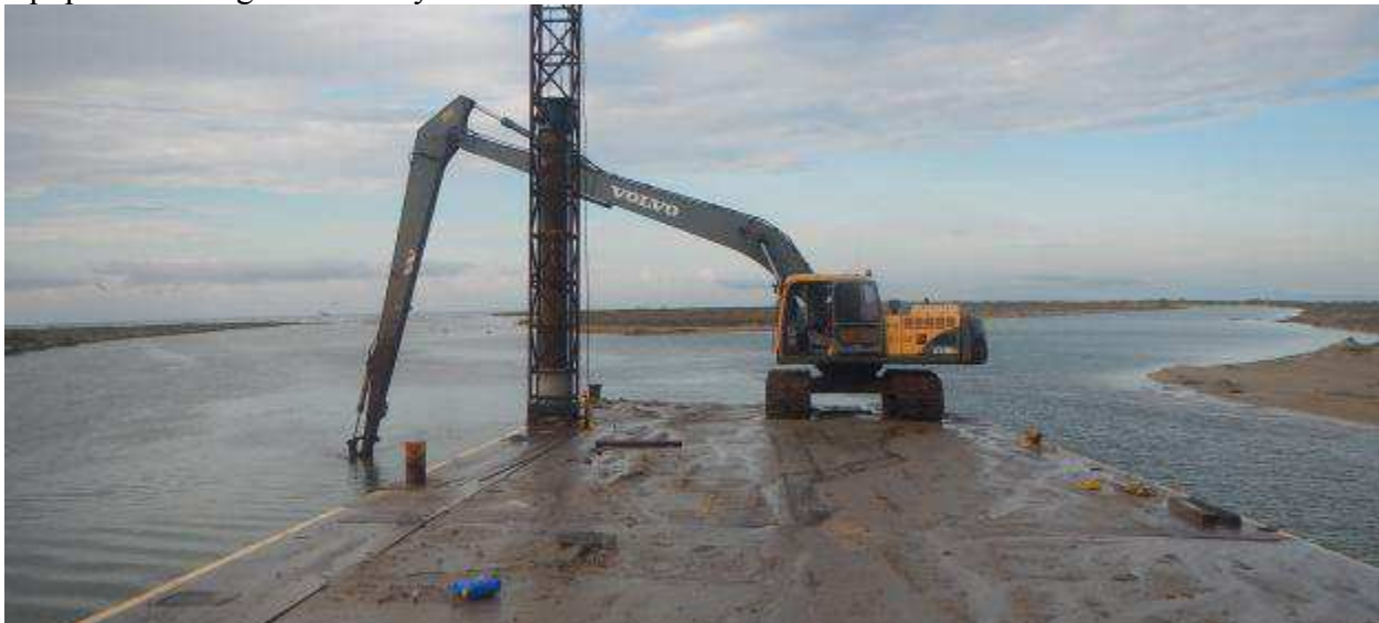
Figure 1. RLB preparing to demobilize equipment through Cedar Bayou
