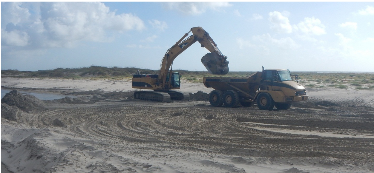
Figure 1. Excavator executing the full cut in Cedar Bayou.
