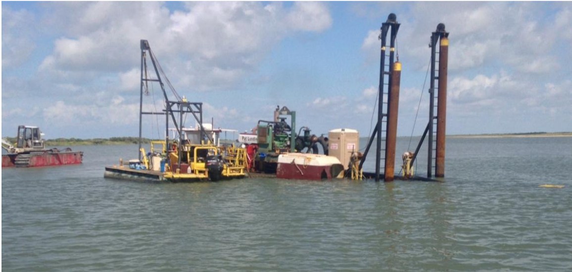
Figure 2. Dredge working in Vinson Slough.
