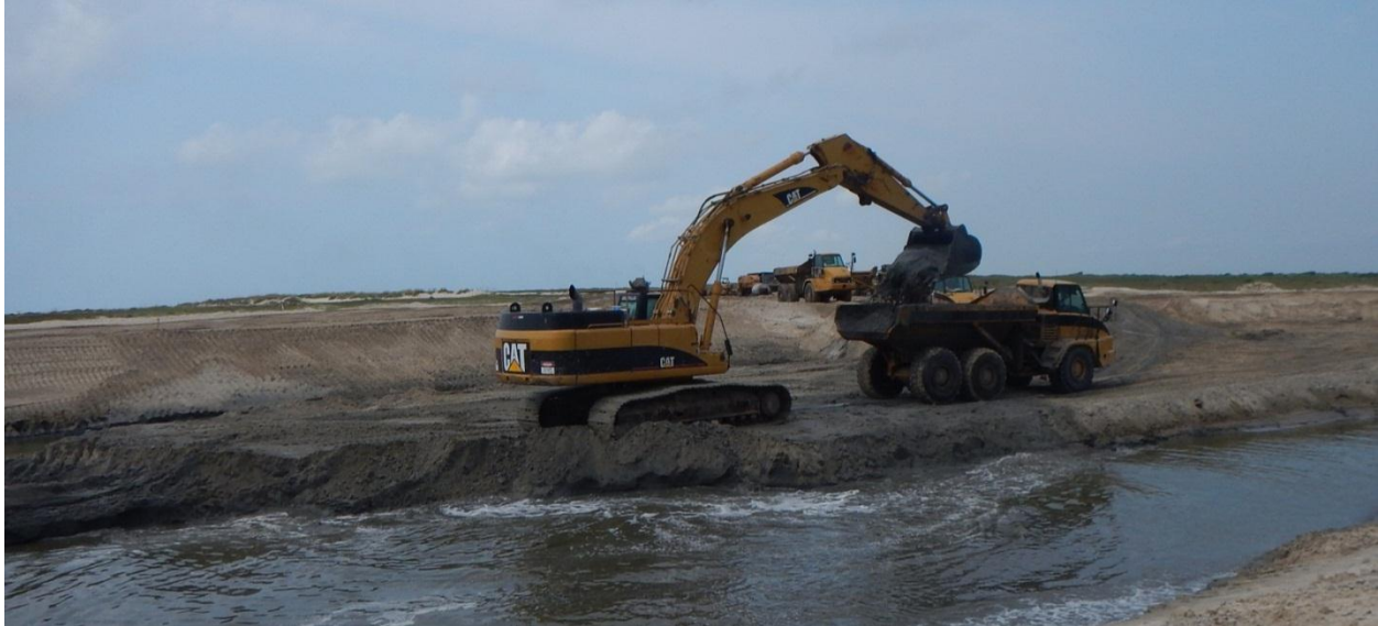
Figure 2. Equipment working in Vinson Slough.
