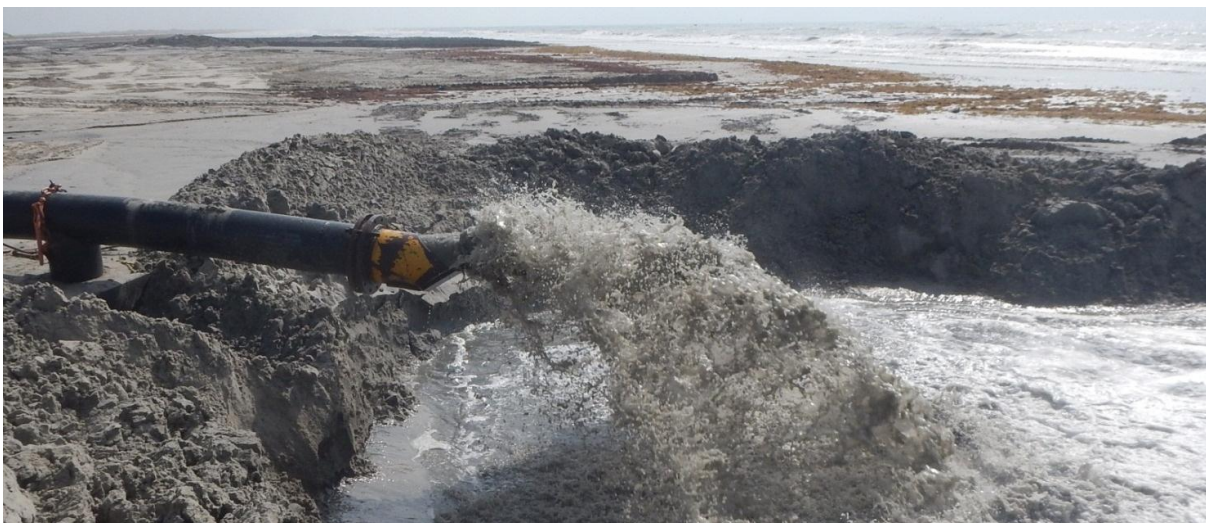
Figure 3. Material flowing out of dredge pipe.
