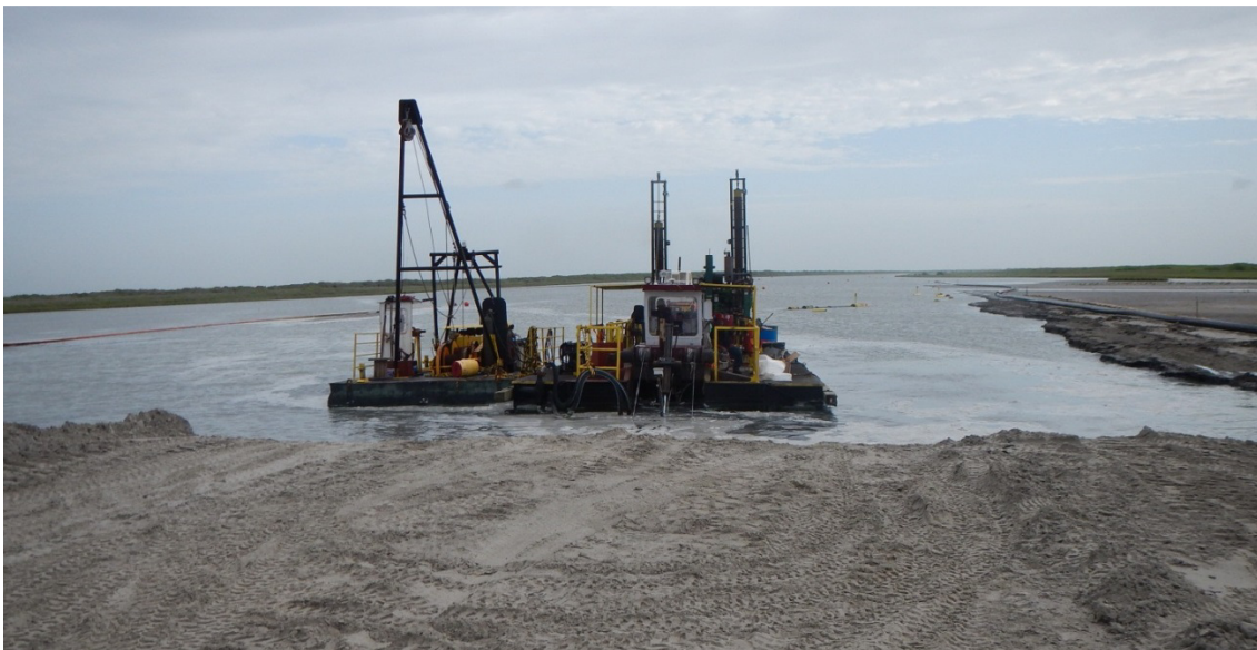
Figure 1. Hydraulic dredge working in Cedar Bayou.
