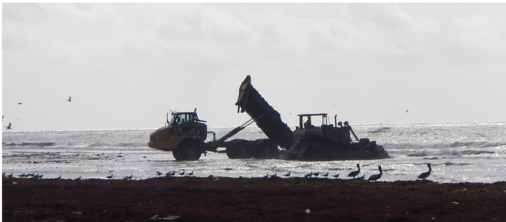
Figure 3. Material being placed and graded in Placement Area 1.
