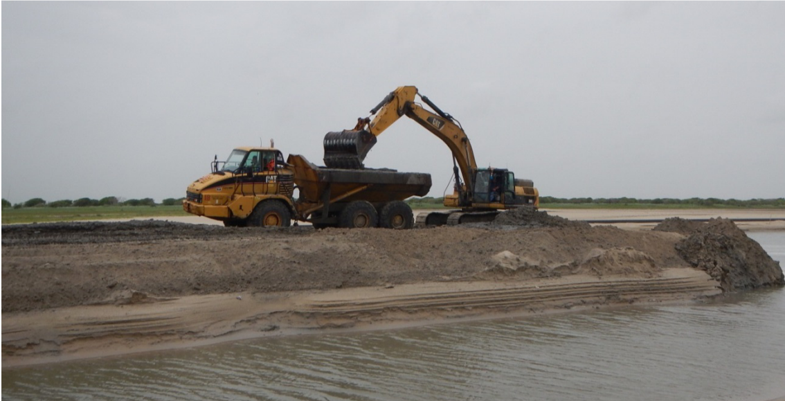
Figure 2. Equipment working in Vinson Slough.
