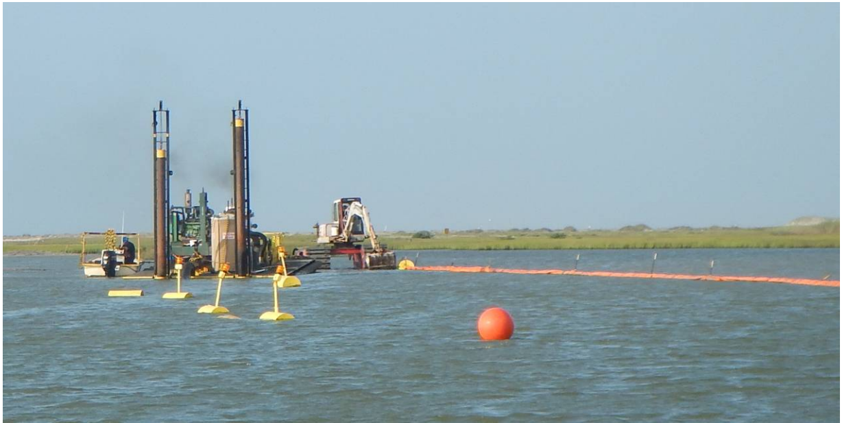
Figure 1. Hydraulic dredge working in Cedar Bayou
