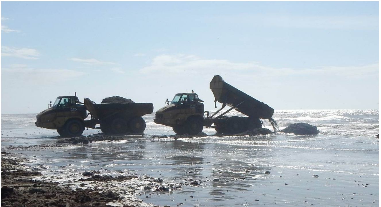
Figure 3. Material hauled from Vinson Slough being deposited onto Placement Area 1.
