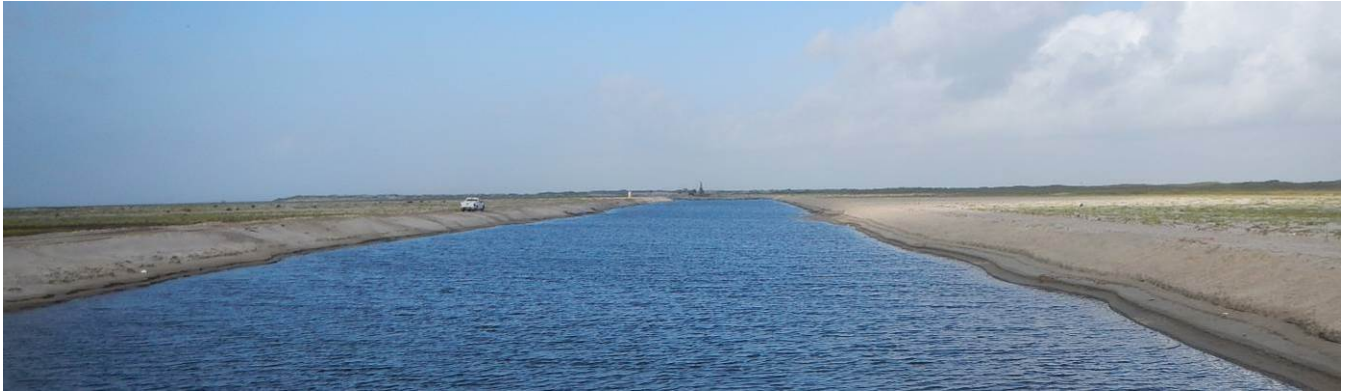
Figure 2. Excavation of Vinson Slough looking east from Cedar Bayou.
