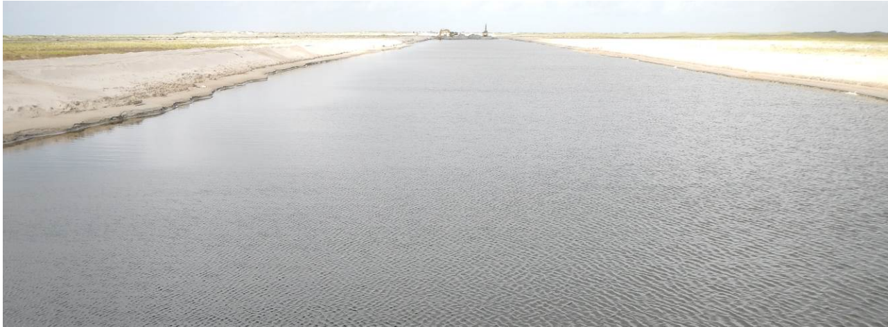
Figure 2. Excavation of Vinson Slough looking east from Cedar Bayou.
