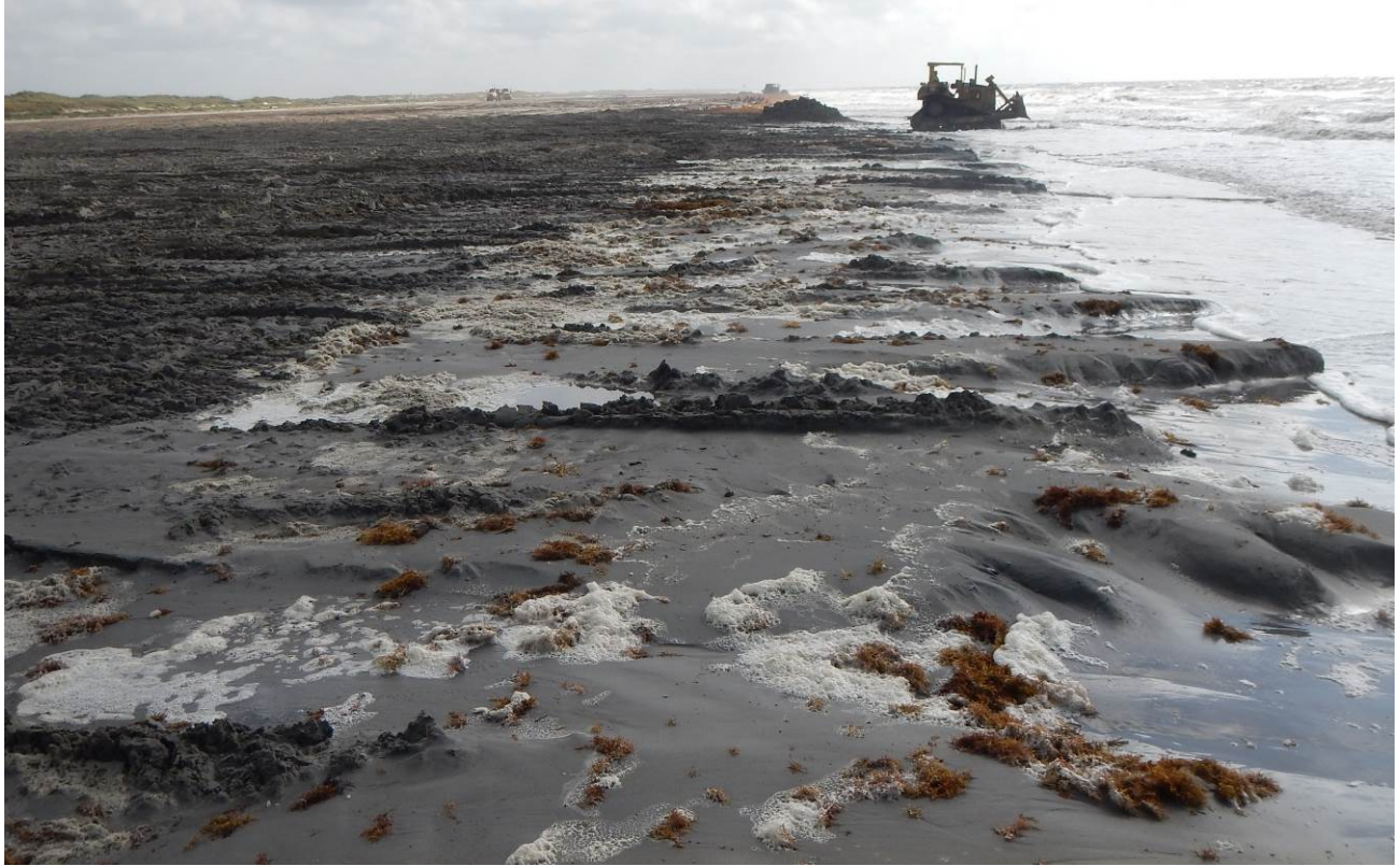
Figure 3. Material hauled from Vinson Slough being graded into Placement Area 1.
