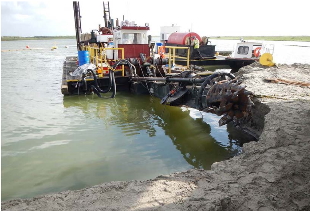
Figure 1. The hydraulic dredge in Cedar Bayou being repaired
