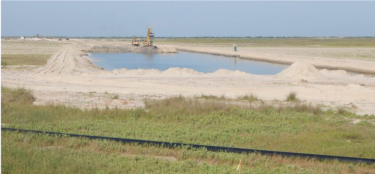
Figure 2. Excavation of Vinson Slough looking east from Cedar Bayou.
