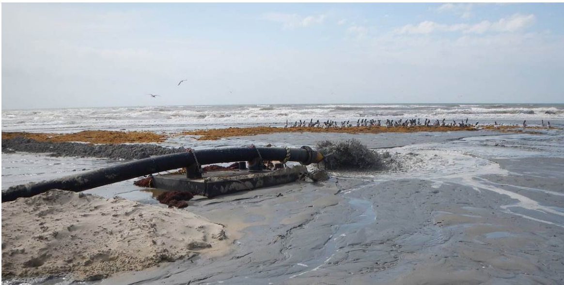
Figure 3. Sand being pumped from Cedar Bayou into Placement Area 1.
