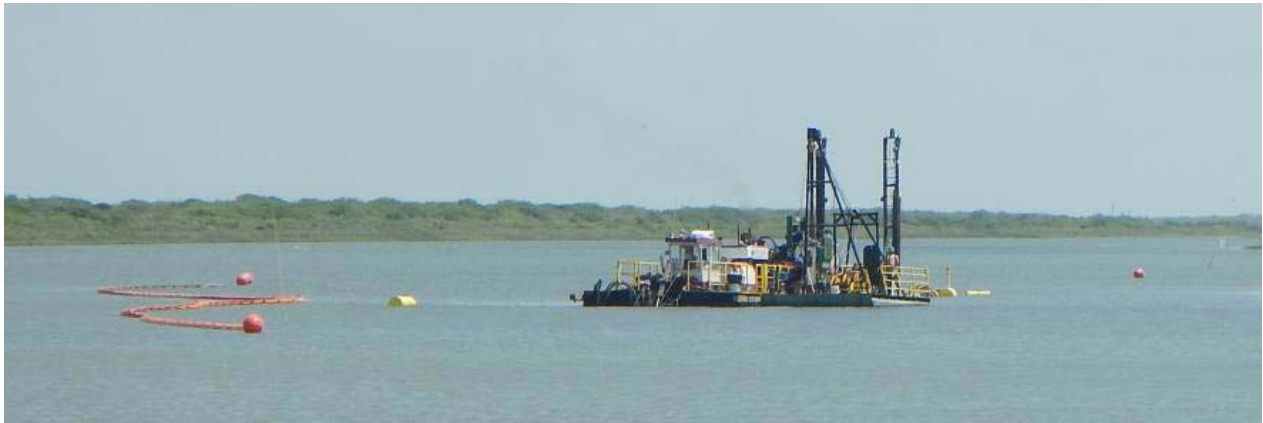
Figure 1. The hydraulic dredge in Cedar Bayou.
