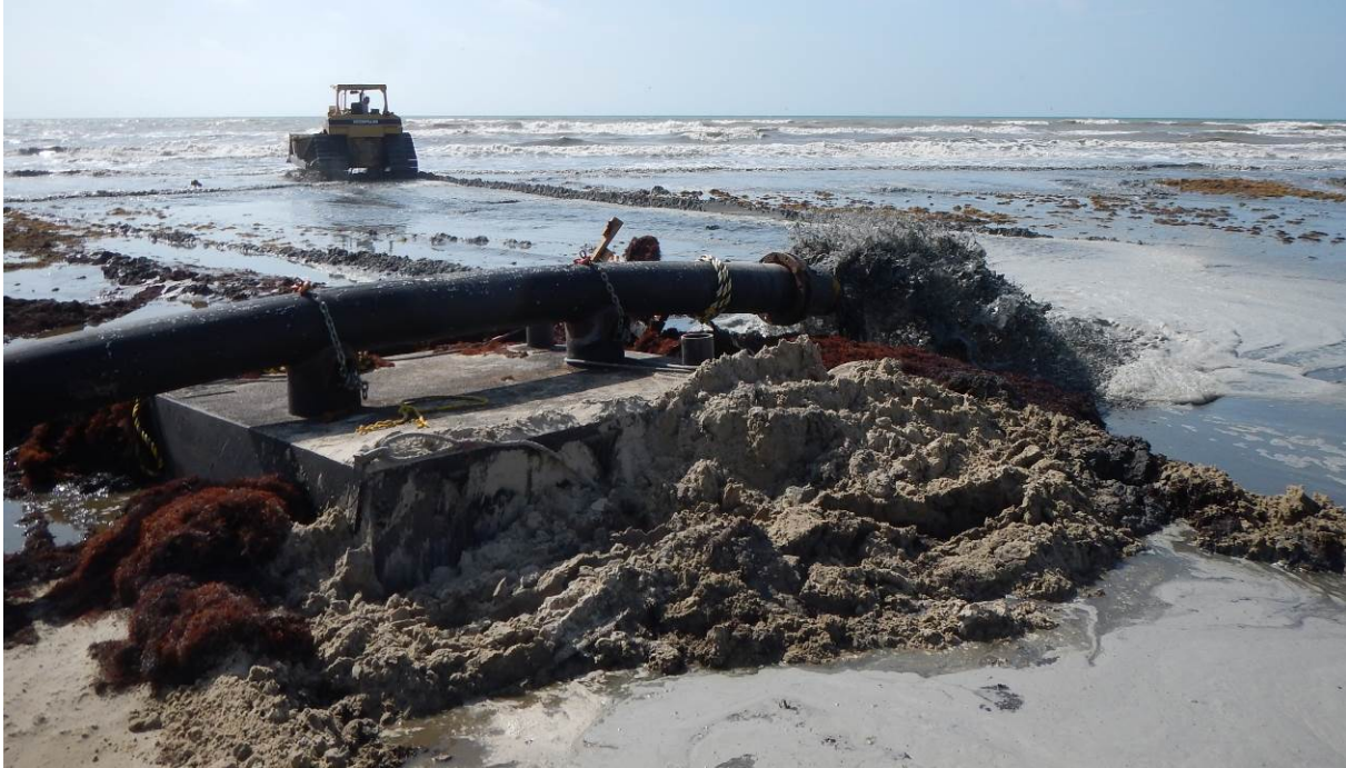
Figure 3. RLB's Dozer blading out material pumped from Cedar Bayou.
