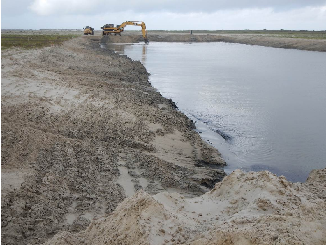
Figure 2. Excavation of Vinson Slough (full channel dimensions shown)
