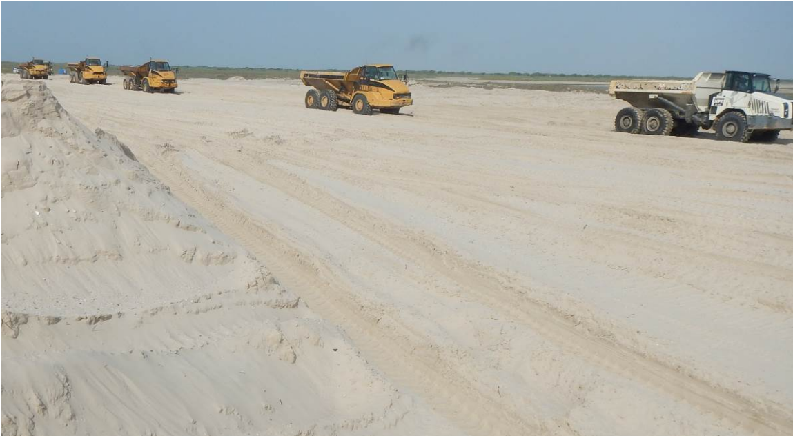
Figure 2. Empty off-road trucks making their way to the spoil pile.
