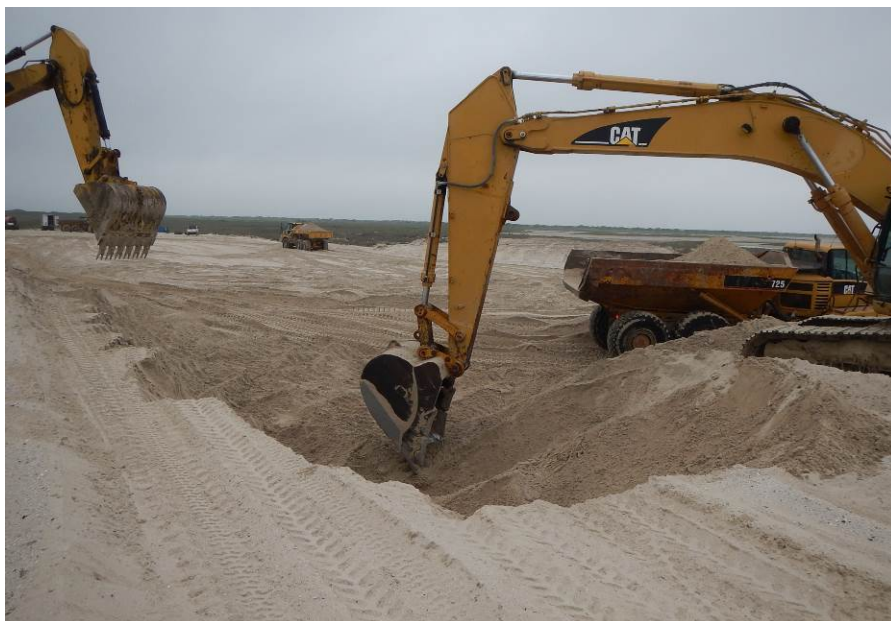
Figure 3. Excavators removing sand from the spoil pile.
