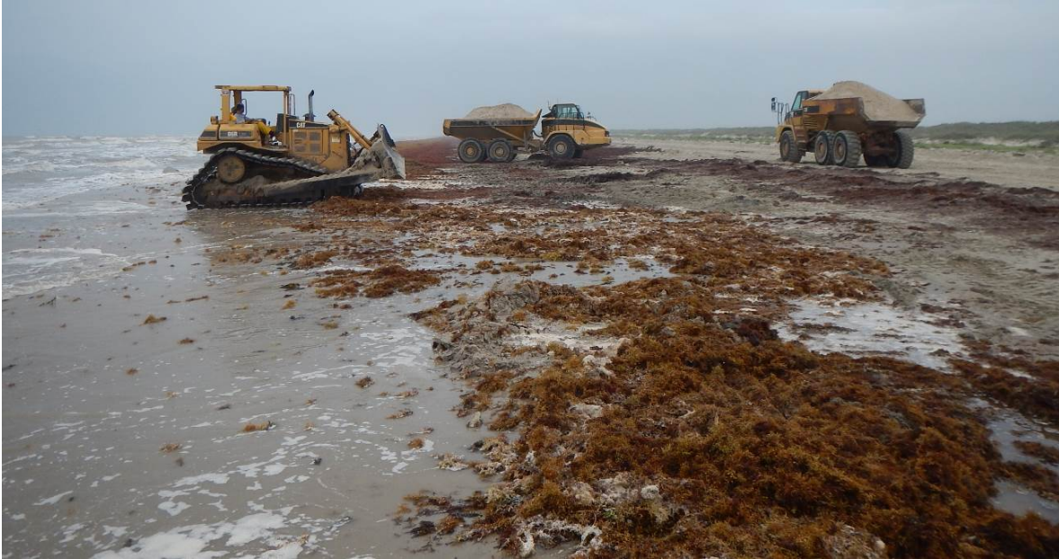
Figure 4. Bulldozer preparing to grade dumped sand in to Placement Area 1.
