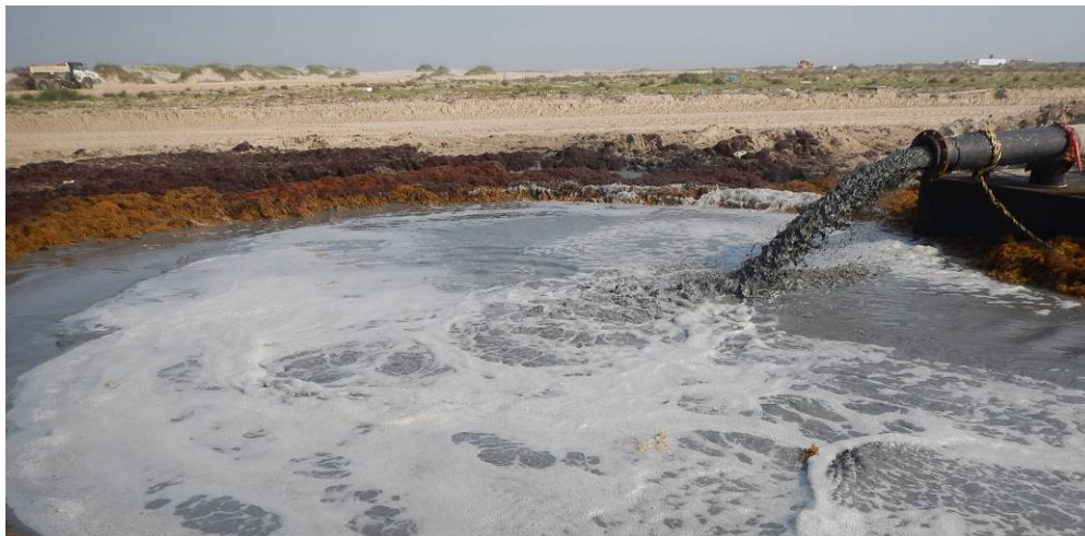
Figure 5. Hydraulic dredge pipeline discharging into Placement Area 1.
